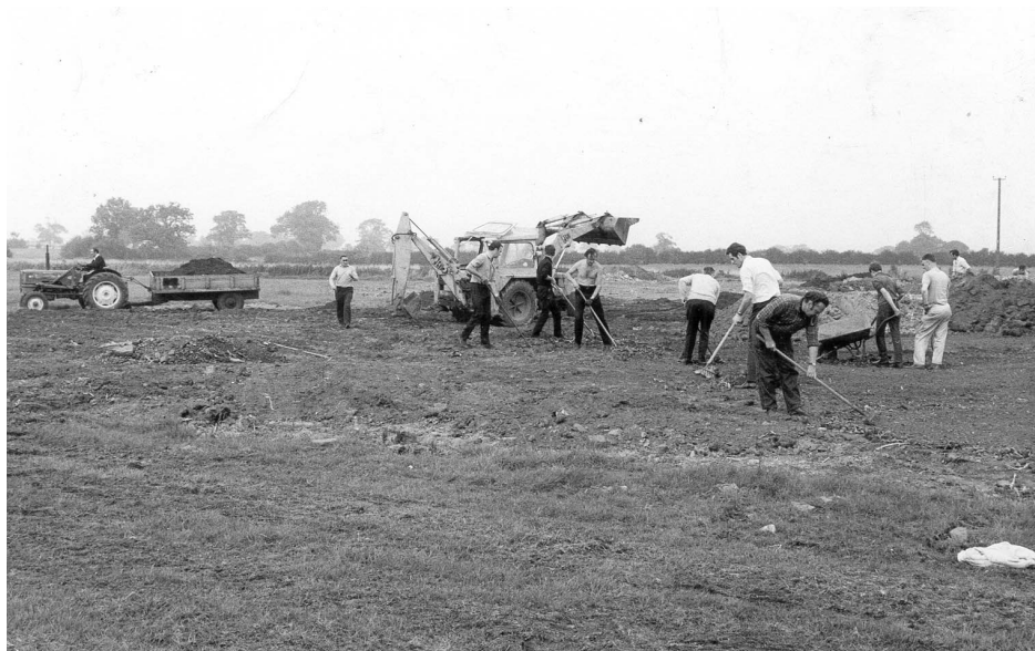
During the autumn of 1970 one thousand tons of topsoil were tipped to raise the level of the ground. On 26 September the course was closed and over 100 members turned out to help with the construction work.
